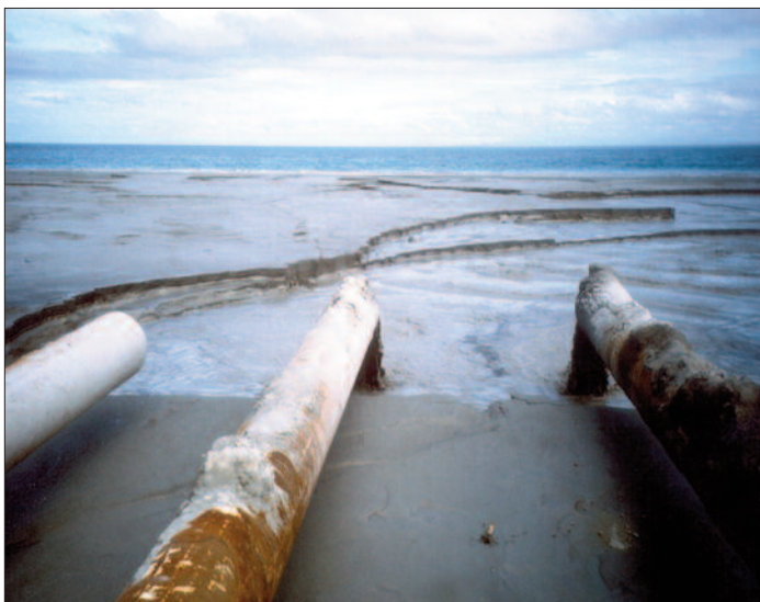
Untreated mine waste dumped into Calancan Bay. Catherine Coumans photo.
