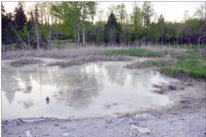
Uncontained contaminated runoff at the abandoned Timminco magnesium mining and processing facility near Renfrew, Ontario. R. Hart photo.
