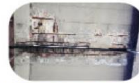
CONCRETE SPALLS
